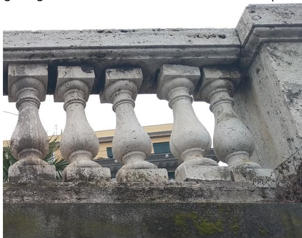
Figura 12 Balaustra in travertino
